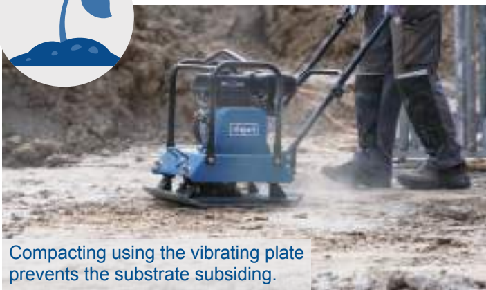
The HP2200s is also suitable for compacting different materials.
