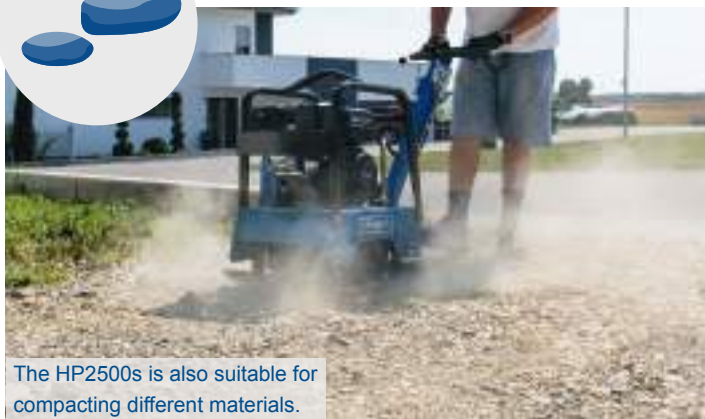
Thanks to the rubber mat, even paving work can be carried out.
