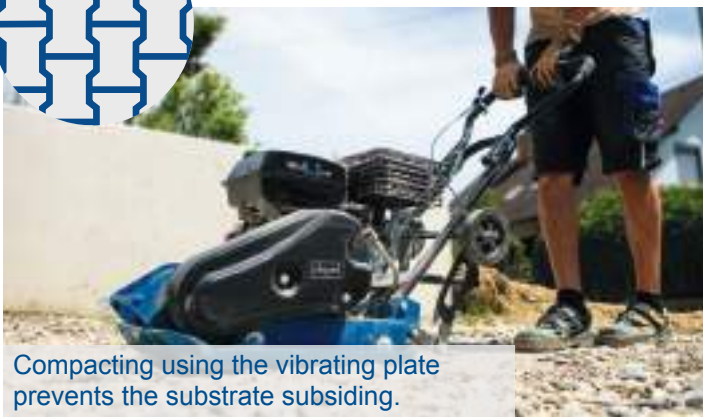
The HP2300s is also suitable for compacting different materials.
